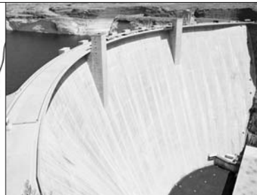
Figure 8.33 Glen Canyon dam in Arizona
