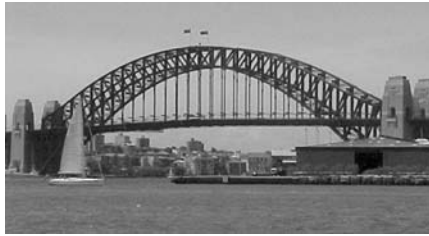
Figure 8.35 Sydney Harbour Bridge
