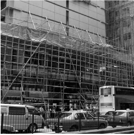
Figure 4.10 Bamboo scaffolding on a building in Hong Kong
